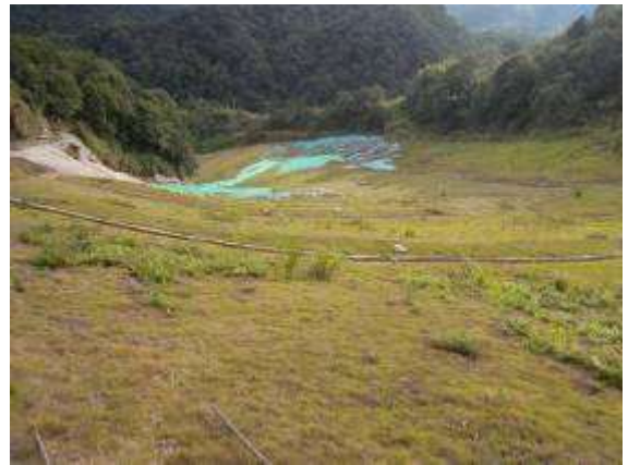
3#尾矿库植被及排水沟 (2017.10.18)
