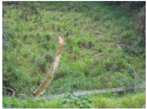
3#尾矿库植被及排水沟 (2017.10.18)
