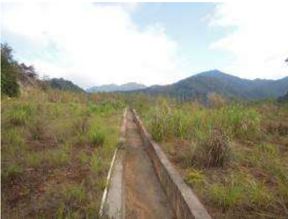
3#尾矿库植被及排水沟 (2017.10.18)
