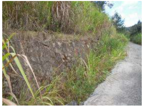
边坡底部挡墙 (2017.10.18)
